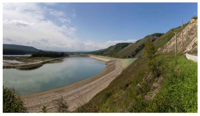
We've built a stability berm at the eastern end of the Lynx Creek segment of Highway 29, in preparation for reservoir filling. See more construction photos in our gallery.
