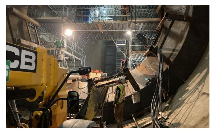
To prepare for reservoir filling, we're installing four large rings inside the second diversion tunnel. These rings will help restrict water flow when we reopen the tunnel. Learn more about tunnel conversion.
