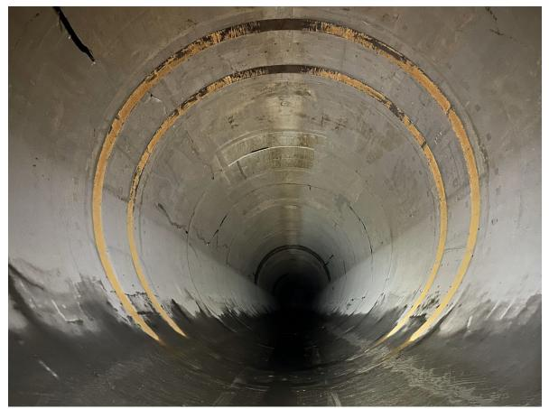
One of two tunnels that have been diverting the Peace River has been closed and water has been pumped out. One of the four large rings will be installed here. This is an important step to prepare for reservoir filling as early as this fall. See more photos in <u>our gallery</u>.
