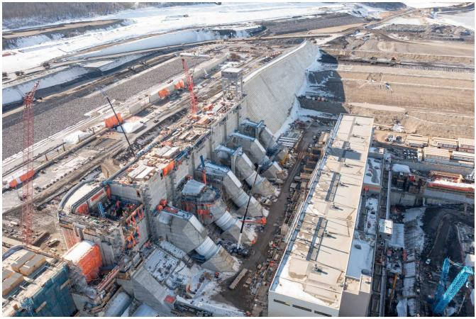
When the Site C dam is in operation, water will flow down the approach channel on the left, through six giant pipes called the penstocks, and into the powerhouse to generate electricity. See more photos in <u>our gallery</u>.
