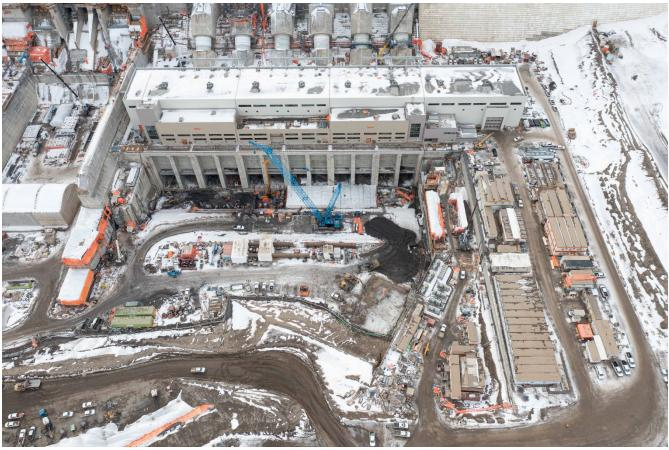
The tailrace, where water will exit the dam after turning turbines inside the powerhouse. See more photos in <u>our gallery</u>.
