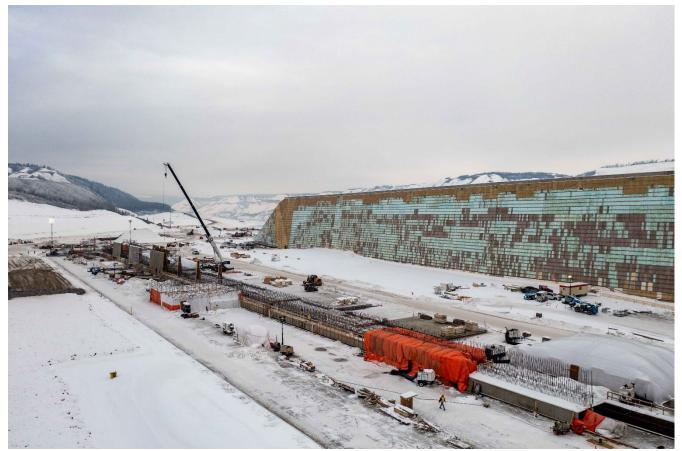
Under heated tarps, concrete cures for the centre wall of the Site C approach channel. Further back, crews install formwork and reinforce steel. See more photos in <u>our gallery</u>.
