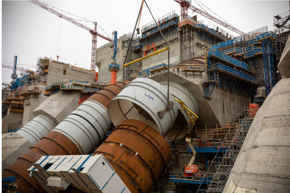
Figure A-14 The Last Penstock Segment is Lowered into Position (June 2022)
