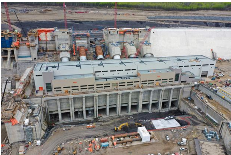
Figure A-10 The Powerhouse and Operation Building are Substantially Complete, with Foundation Enhancements Work Ongoing in Front of the Tailrace (May 2022)
