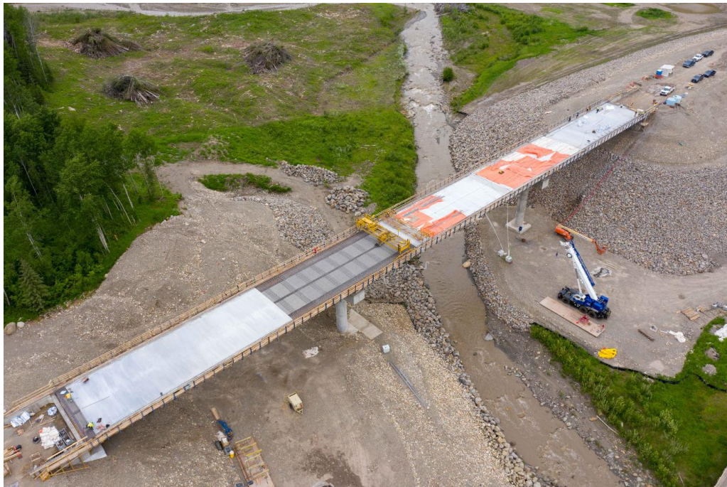
Figure A-15 Lynx Creek Bridge Before the Final Concrete Pour (June 2022)
