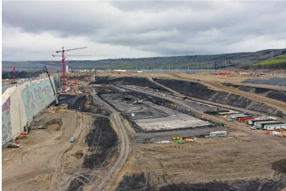
Figure A-9 Ongoing Construction of the Approach Channel (May 2022)
