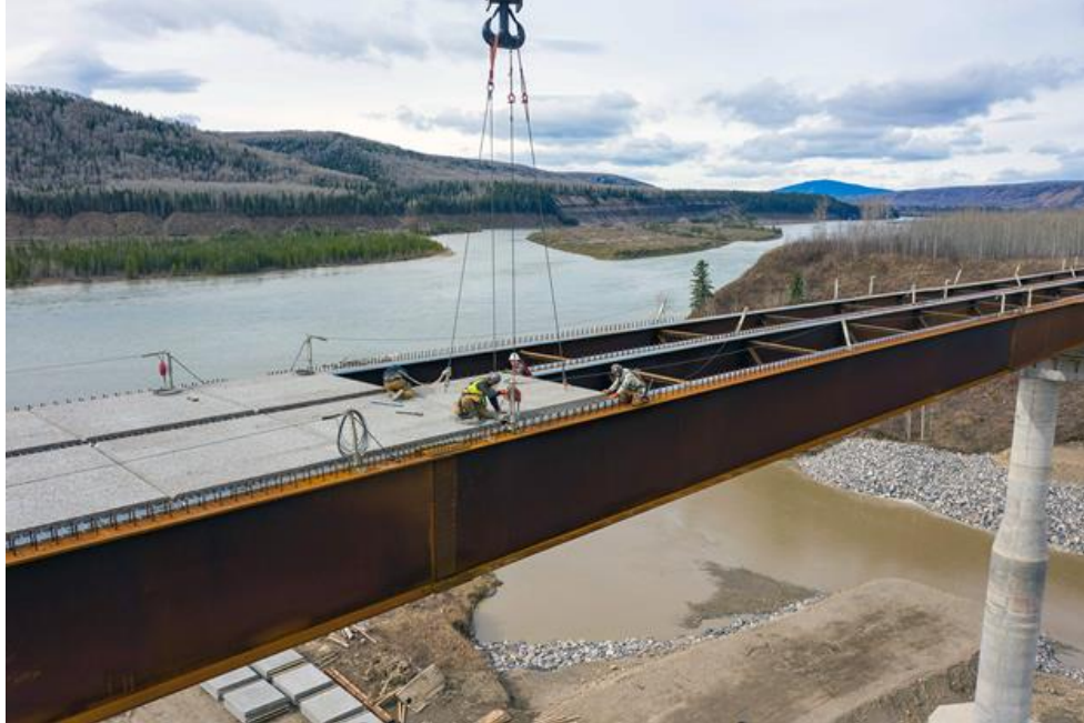
Figure A-7 Pre-Cast Concrete Panels are Moved into Position on the Farrell Creek Bridge at The Highway 29 Realignment (May 2022)
