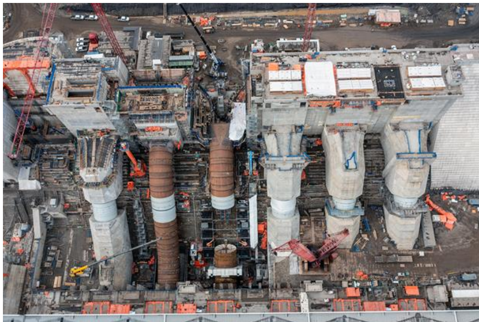
Figure A-6 Penstock Units 1 Through 6 (Unit 1 on the Right) in Varying Stages of Construction (May 2022)
