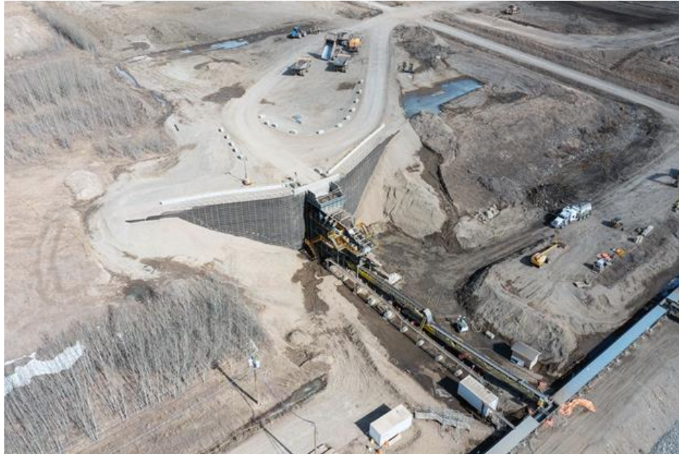
Figure A-3 The Hopper and Feeder are The Primary Supply Loading Point for the Conveyor that Transports Glacial Till from the 85 th Ave Industrial Lands to Site C (April 2022)
