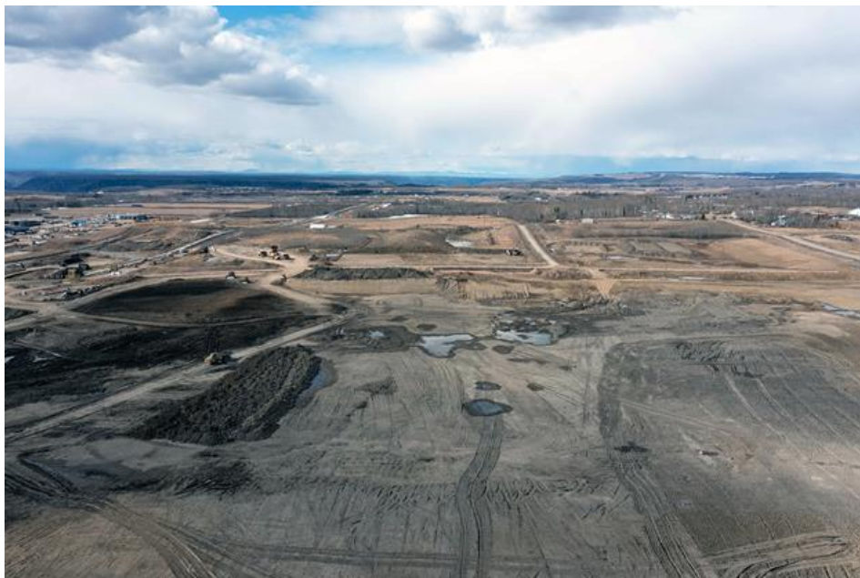
Figure A-2 A West Facing View Over the 85 th Ave Industrial Lands Where Glacial Till is Excavated to Build the Site C Dam (April 2022)
