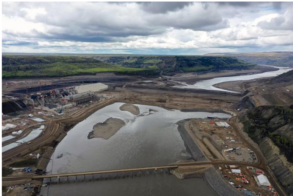
Figure A-8 An Upstream View of the Powerhouse and Generating Station, with Laydown Areas, Temporary Fishway and Outlet Portals (May 2022)
