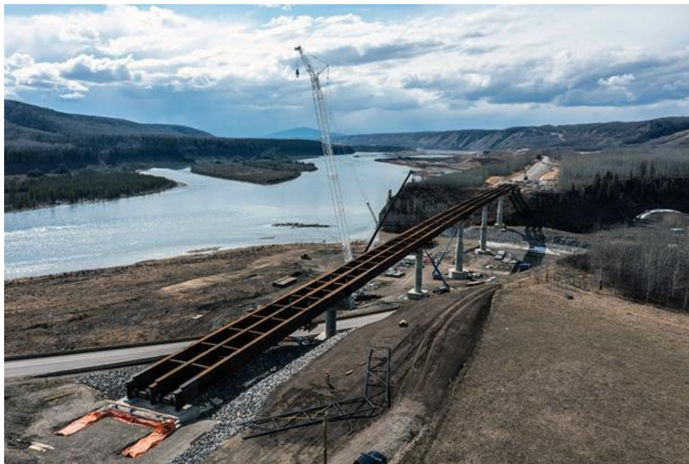
Figure A-4 Steel Installation is Complete on the Farrell Creek Bridge Deck (April 2022)
