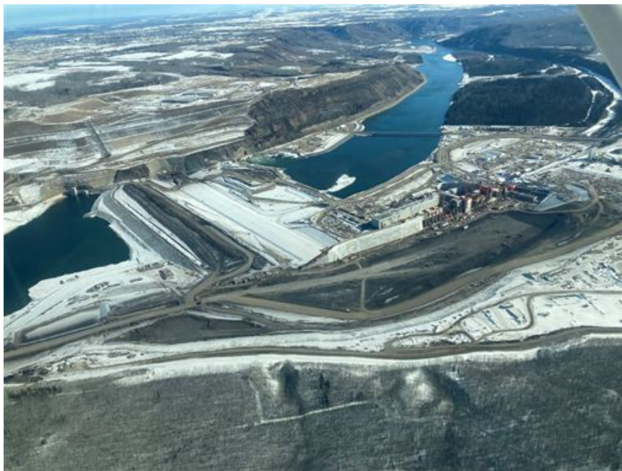
Progress Photo, March 2022
