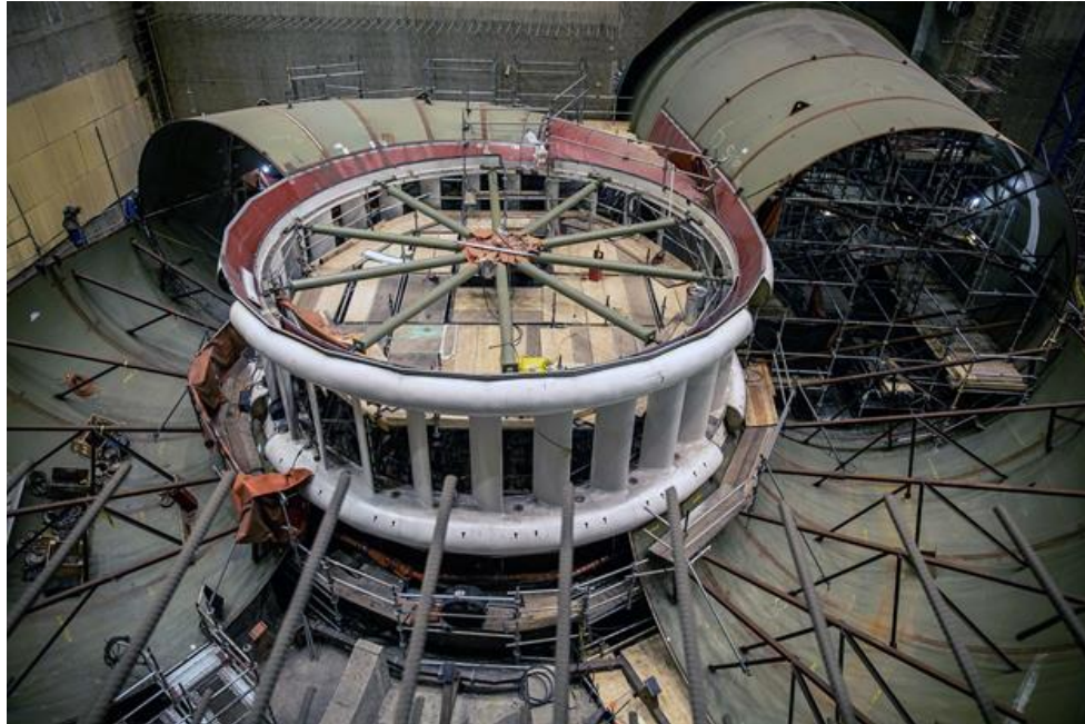
Figure A-1 Ongoing assembly of the Unit 6 Spiral Case and Stay Ring (April 2022)
