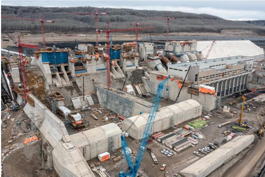
Figure A-5 Spillways, Penstocks, Powerhouse and Operations Building (May 2022)
