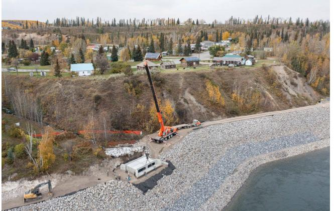
Crews install a concrete box culvert as part of construction of the Hudson's Hope shoreline protection berm. For more photos, see the image gallery.
