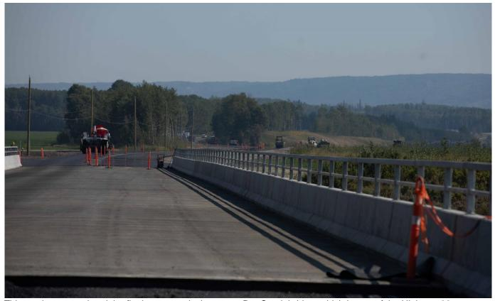
This week we completed the final concrete deck pour on Dry Creek bridge, which is part of the Highway 29 realignment. See more photos in the <u>image gallery</u>.
