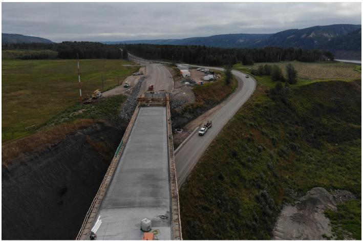
Crews complete one of the final concrete deck pours on Farrell Creek bridge, as part of the Highway 29 realignment. See more photos in the <u>image gallery</u>.
