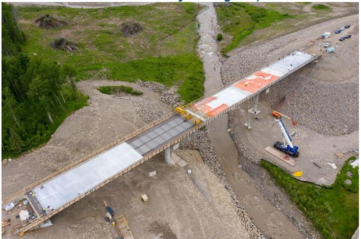
The final concrete deck pour for Lynx Creek bridge as part of the Highway 29 realignment. See more photos in the <u>image gallery</u>.
