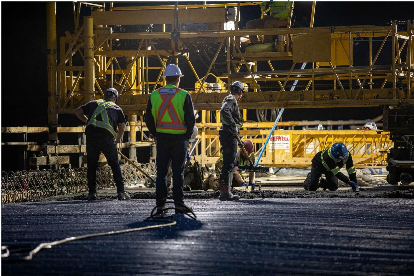
Crews work overnight to complete a concrete pour on the Lynx Creek Bridge deck, as part of the Highway 29 realignment. See more photos in the [image gallery](#).
