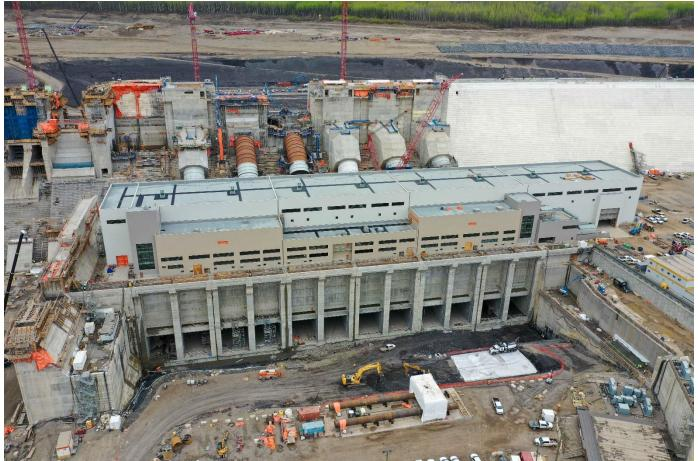
The powerhouse and operation building are substantially complete, with ongoing foundation enhancement work happening near the tailrace. See more photos in the <u>image gallery</u>.
