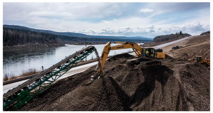
A rock crusher is turning aggregate into finer material for Highway 29 road work at Lynx Creek. See more photos in the <u>image gallery</u>.
