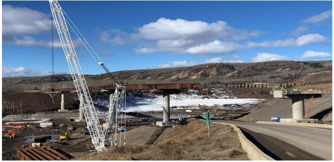
Crews installed steel girders for the Farrell Creek Bridge, part of the Highway 29 realignment. See more photos in the <u>image gallery</u>.
