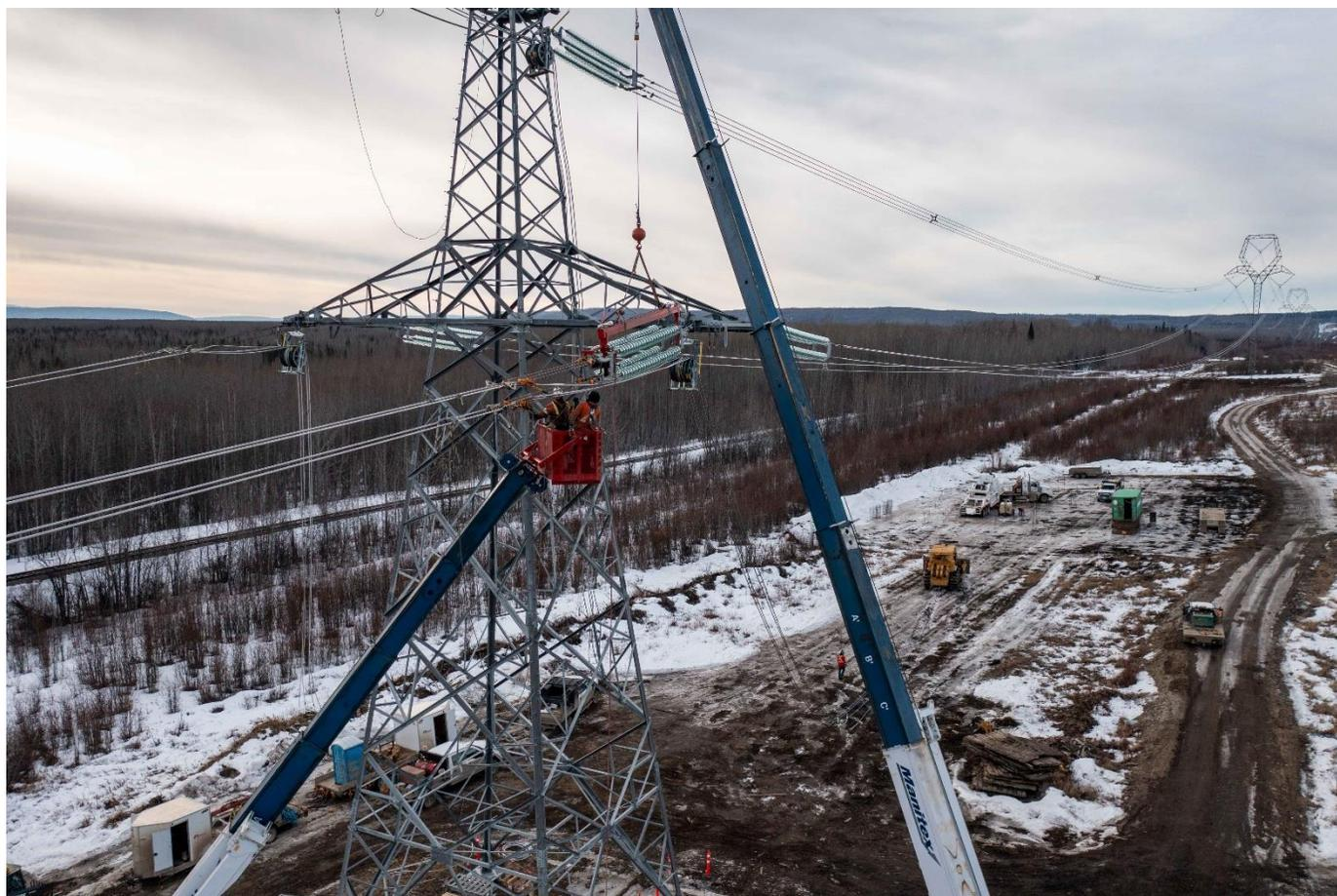
Crews are attaching the last conductors to complete the second of two 500 kv transmission lines, which is expected to be energized in the coming weeks. More photos in the [image gallery](#).
