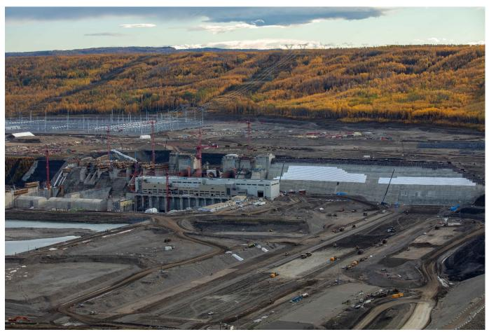
A view of the dam core trench, dam buttress, powerhouse, spillways, and the operational substation in the background. The white cladding material on the dam buttress is insulation that protects the concrete and allows it to cure through the winter. See more project photos in the <a href="magegallery">image gallery</a>.
