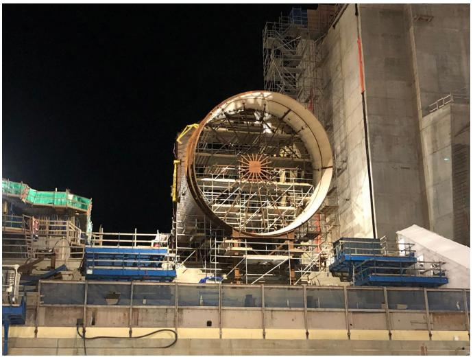
A penstock section for the unit 4 intake – the last intake to be built. Intake units 2 and 5 are under construction. Units 1 and 3 are substantially complete. See more project photos in the image gallery.
