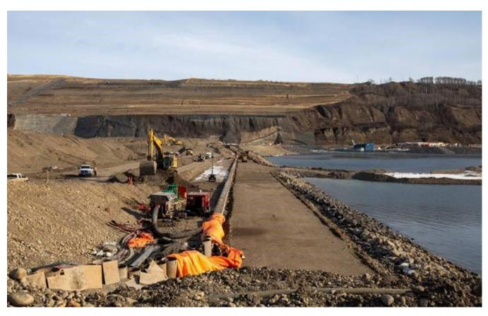
Crews have completed the downstream cofferdam. With both the upstream and downstream cofferdams now complete, crews can begin constructing the earthfill dam. See more project photos in the <u>image gallery</u>.
