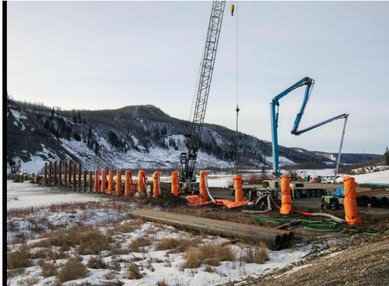
**Figure A-10** An Aerial View of the Moberly River Pile Structure under Construction. This Structure, in Combination with a Debris Boom, will be Used to Capture Debris Floating in the River (February 2020)
