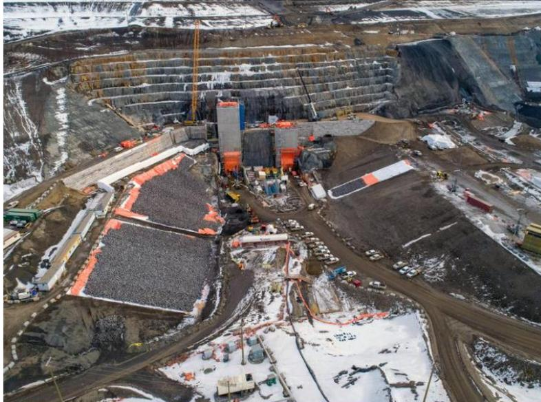
**Figure A-6** Aerial View of the Diversion Tunnel Outlet Portals and the Temporary Fish Passage Facility under Construction (February 2020)
