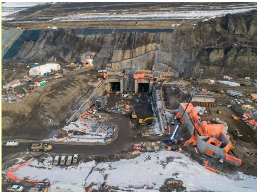
**Figure A-7** Dam Core Trench Excavation on the North Bank is Nearing Completion (February 2020)
