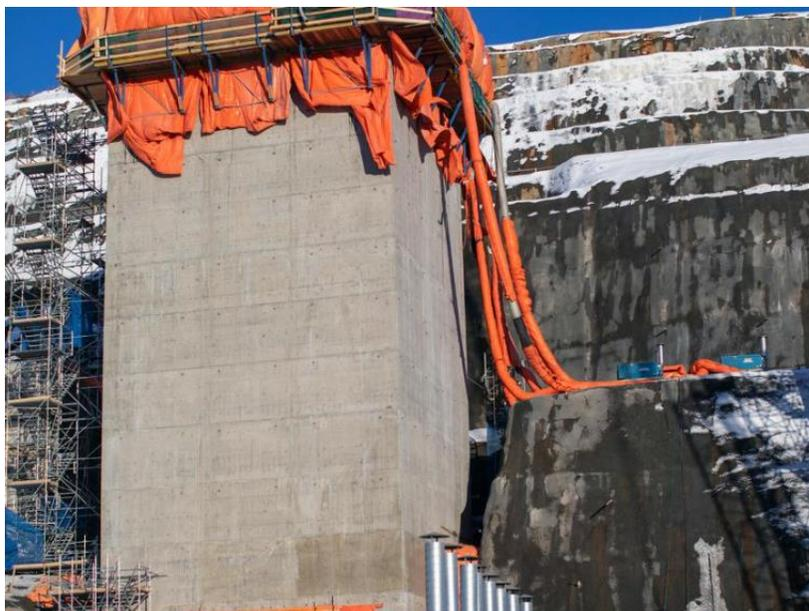
**Figure A-5** Aerial View of the Diversion Tunnel Inlet Portals. The Tower Structures House the Mechanical Gates Required to Control Water Flows into the Tunnels (February 2020)
