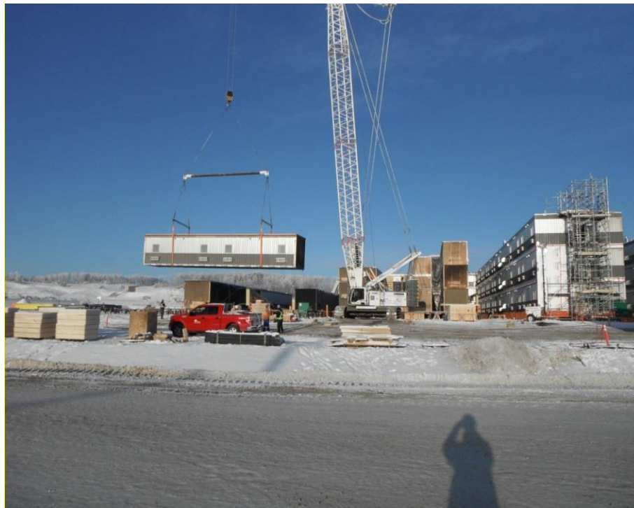
Figure A4 Worker Camp Under Construction
