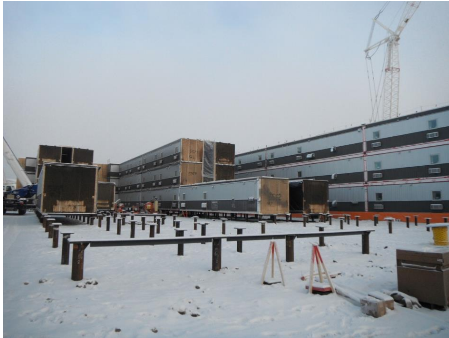
Figure A5 Worker Camp Under Construction
