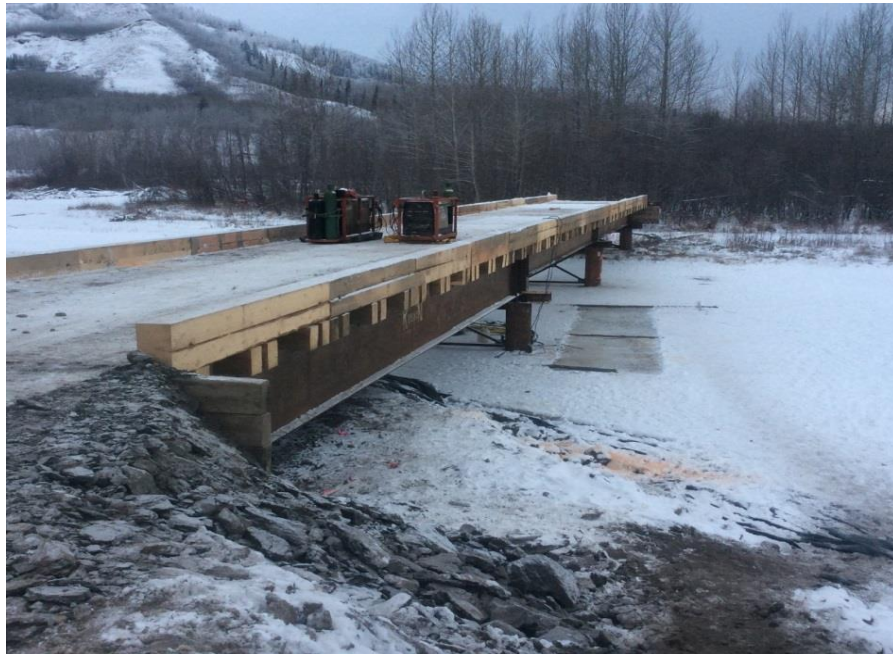
Figure A3 Lower Moberly Bridge
