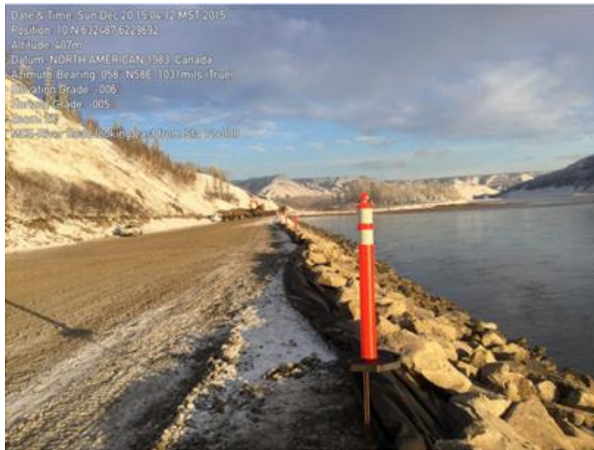
Figure A2 North Bank Site Preparation Looking East Along River Road
