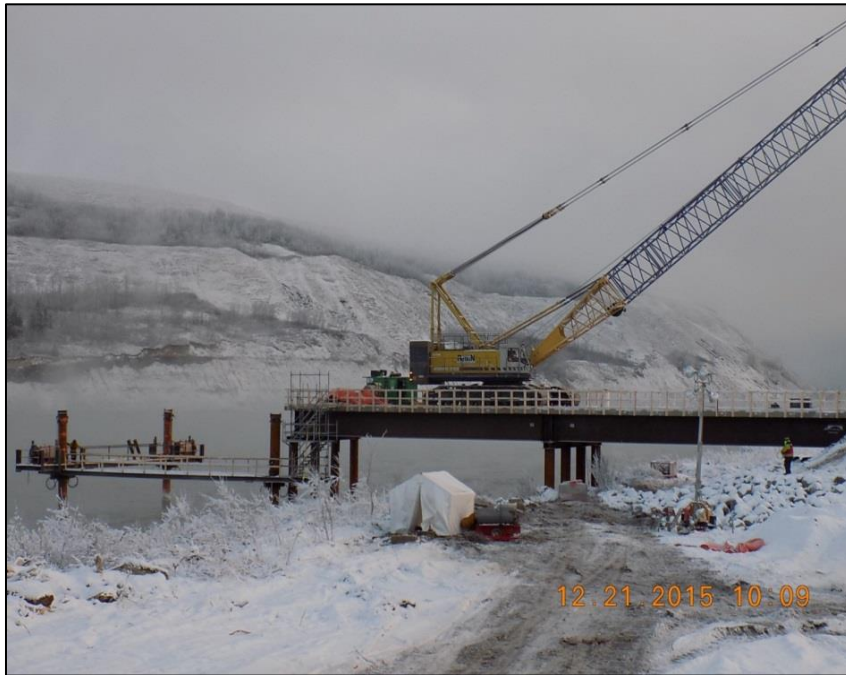
Figure A1 Preparing for Pile Driving for the Construction Bridge
