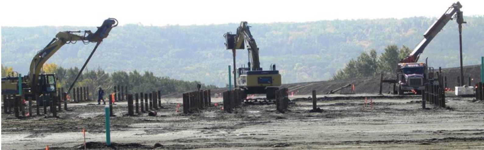
Figure A-4 Worker Camp under Construction: Crews Installing Foundation Piles
