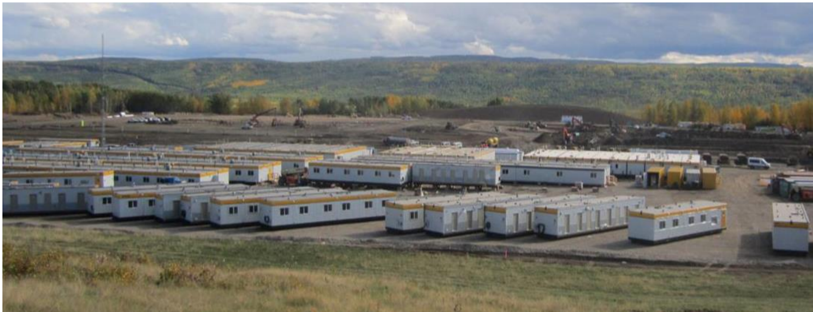
Figure A-3 Temporary Camp in Place, until Main Camp Complete
