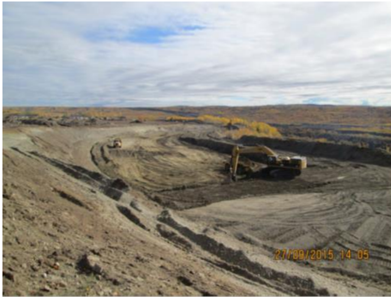
Figure A-1 Excavation Area on the Left Bank
