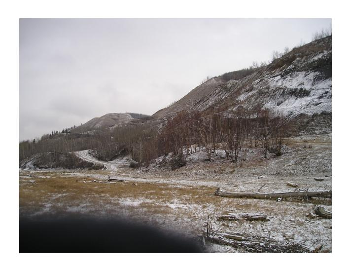
Site C3 – On the toe of the Left abutment looking at the shale outcropping (standing at about Elev.420+/-). Top of the shale is near the top of the proposed dam at Elev. 460+/-.
