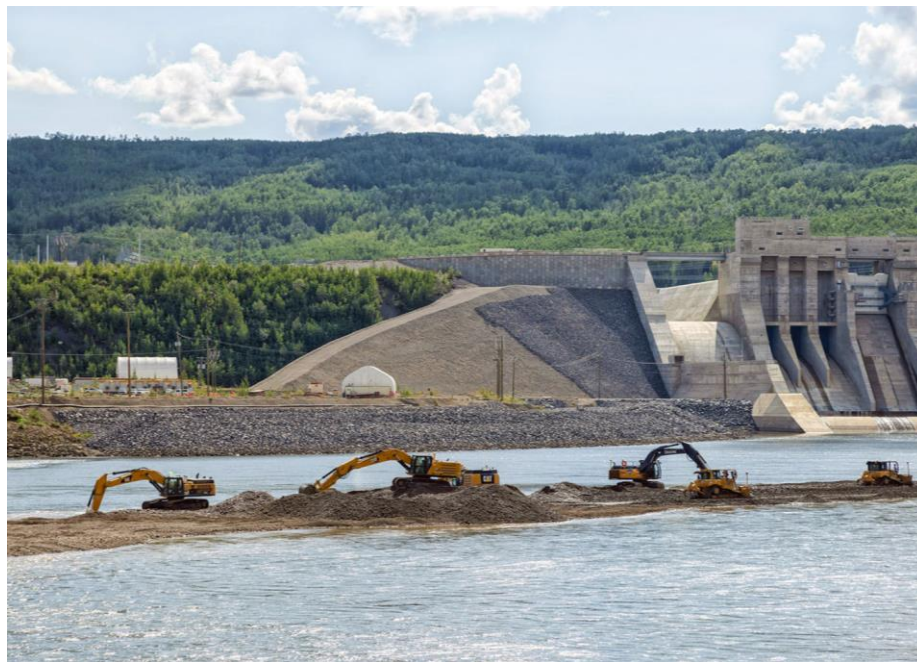
Figure A-8 The excavation of the tailrace area. This excavation also mitigates the potential for fish stranding. (August 2025)
