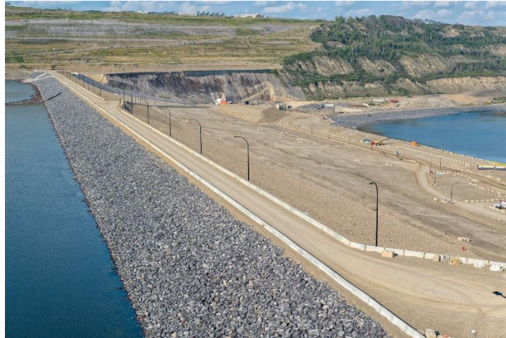
Figure A-3 Looking north along the crest of the earthfill dam. Light standards have now been installed at various locations on the earthfill dam. (July 2025)
