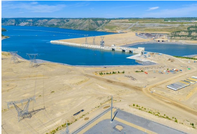
Figure A-5 Looking upstream at the Site C reservoir, the earthfill dam, the approach channel, intakes and spillways. The transmission lines between the powerhouse and substation are in the lower left. (July 2025)
