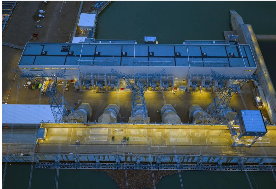
Figure A-7 Aerial view of the Site C intake deck, penstocks, main transformers, and powerhouse. (August 2025)
