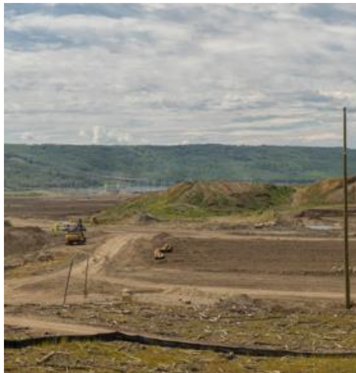
Figure A-16 The eastern edge of the right bank reclamation area. The fencing shown in the foreground is used to prevent amphibians from entering the construction area. (July 2025)
