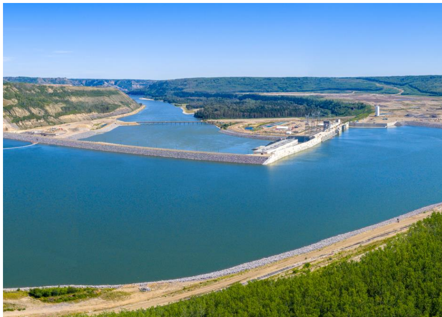
Figure A-2 Looking downstream with the Site C earthfill dam (left) and the approach channel (right). Permanent debris booms continue to direct debris to the north (left) bank away from the approach channel. (July 2025)
