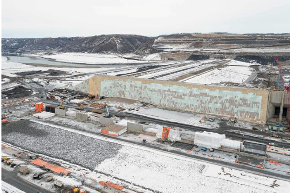
Figure A-5 Construction of the approach channel wall | February 2023
