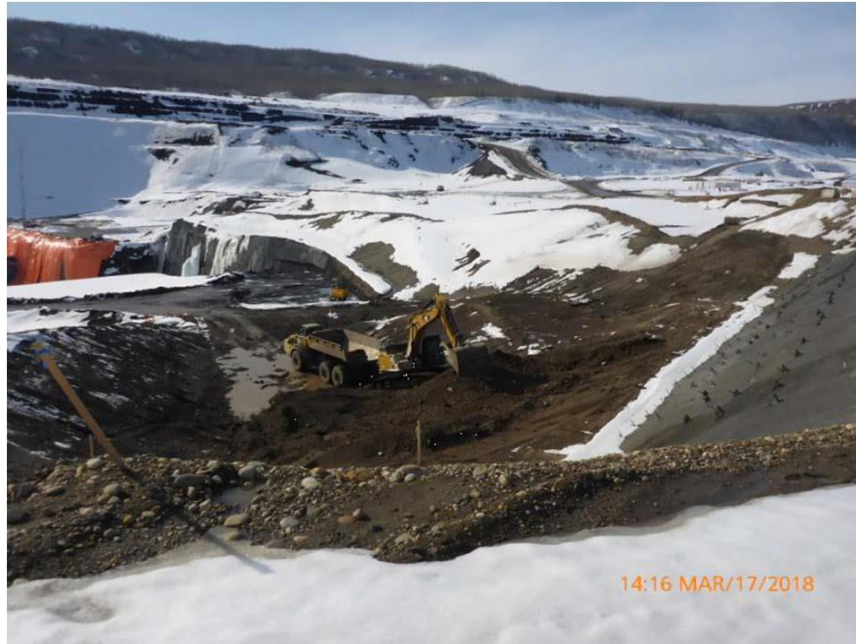
Figure A-7 Tailrace Wall Excavation. Photo taken March 17, 2018.
