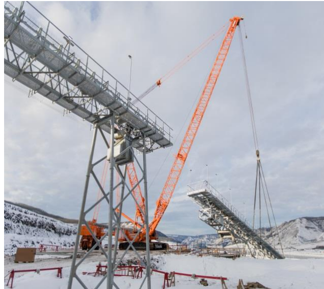
Figure A-1 Installing Conveyor Equipment at the Approach Channel and Powerhouse Buttress on the South Bank. Photo taken January 19, 2018.
