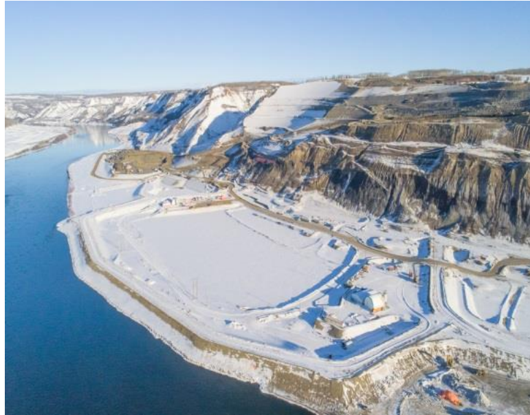
Figure A-3 Aerial View of the North Bank with Cofferdam and Excavation, Facing Northwest. Photo taken February 28, 2018.
