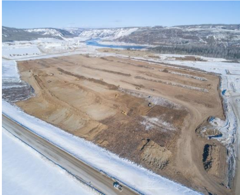
Figure A-5 Aerial View of the South Bank, with Generating Station and Spillways Aggregate Area. Photo taken February 28, 2018.
