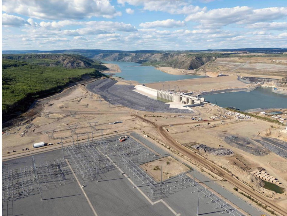
Figure A-6 The Site C dam site | August 2024
