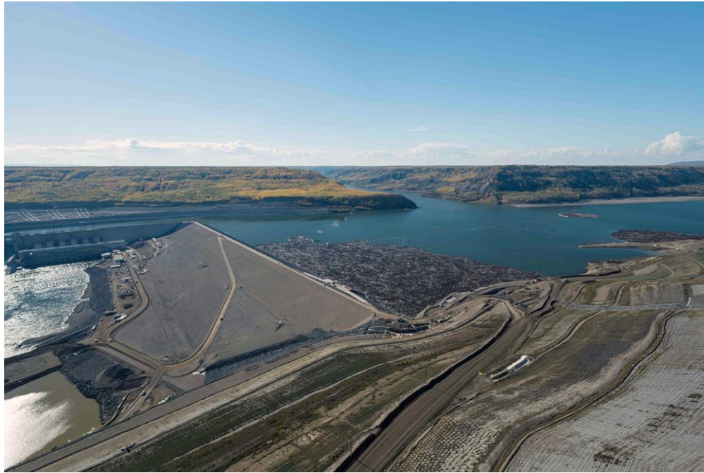
Figure A-10 The dam site and the collection and removal of wood debris during reservoir filling | September 29, 2024
