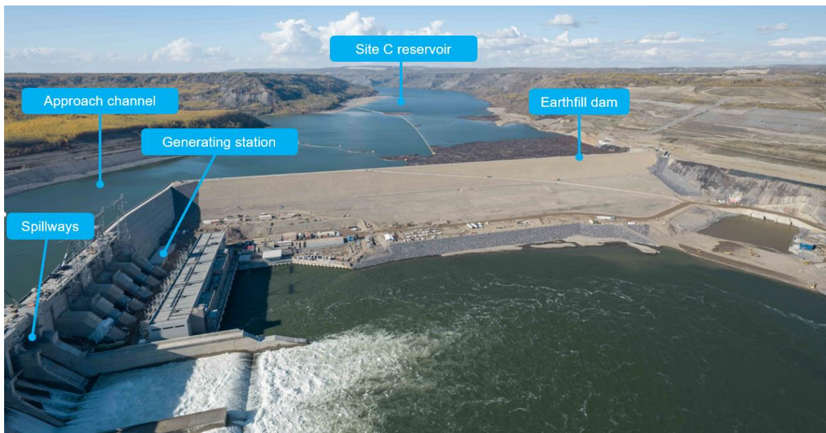
8 Figure 1 The Site C Dam Site (as seen in 9 September 2024).
