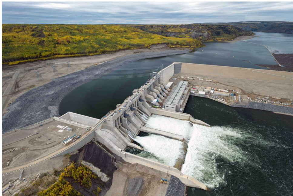
Figure A-11 Dam site | September 29, 2024
