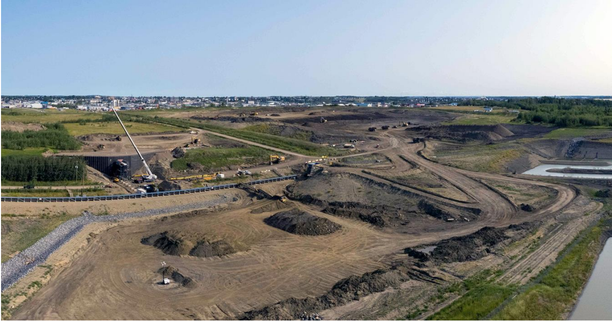
Figure A-10 Crews in the dam core trench are busy placing till, filters and aggregates (September 2021)
