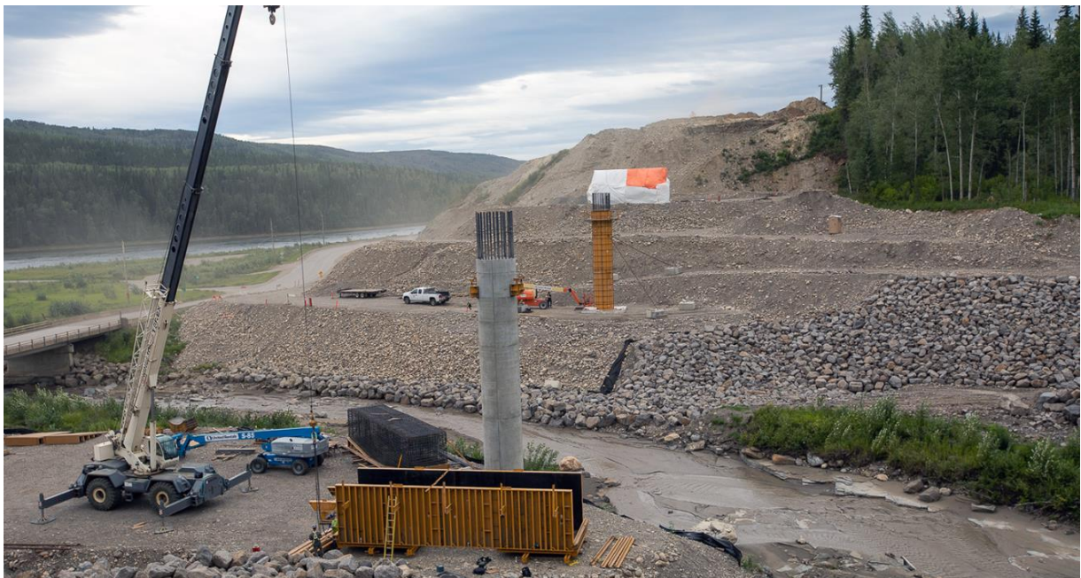
Figure A-8 Construction of the concrete piers for the Lynx Creek bridge along Highway 29 (August 2021)
