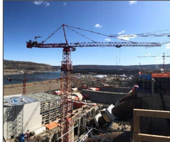
Figure 1 Sir Pix-A-Lot, a Potain MD 3200 tower crane supports construction of the Site C penstocks.
