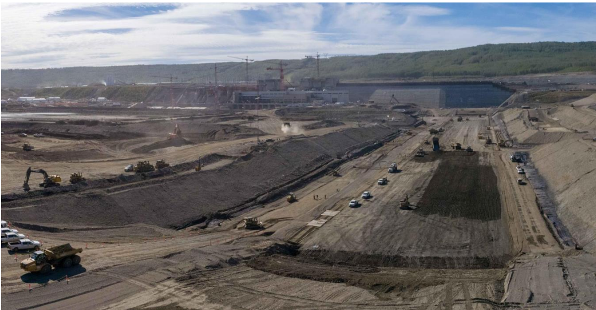
Figure A-10 Crews in the dam core trench are busy placing till, filters and aggregates (September 2021)
