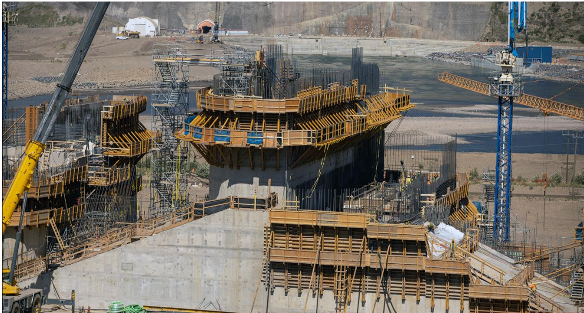
Figure A-7 Construction is ongoing on the spillway headworks centre pier at bay 2 and 3 (August 2021)
