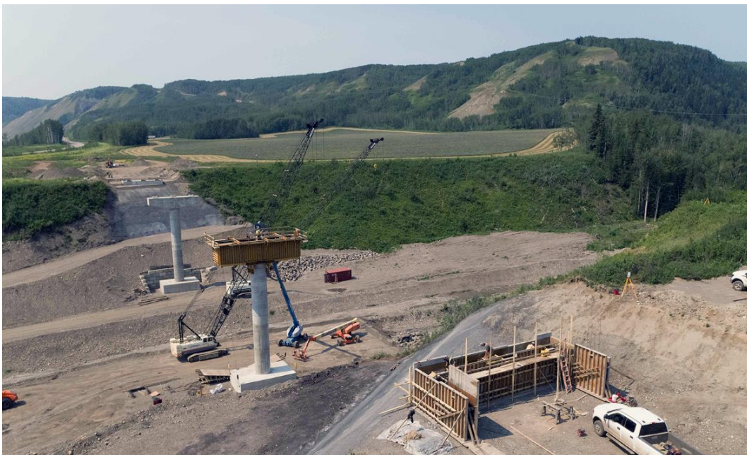
Figure A-2 Bridge formwork is under construction at the Dry Creek section of Highway 29 (July 2021)
