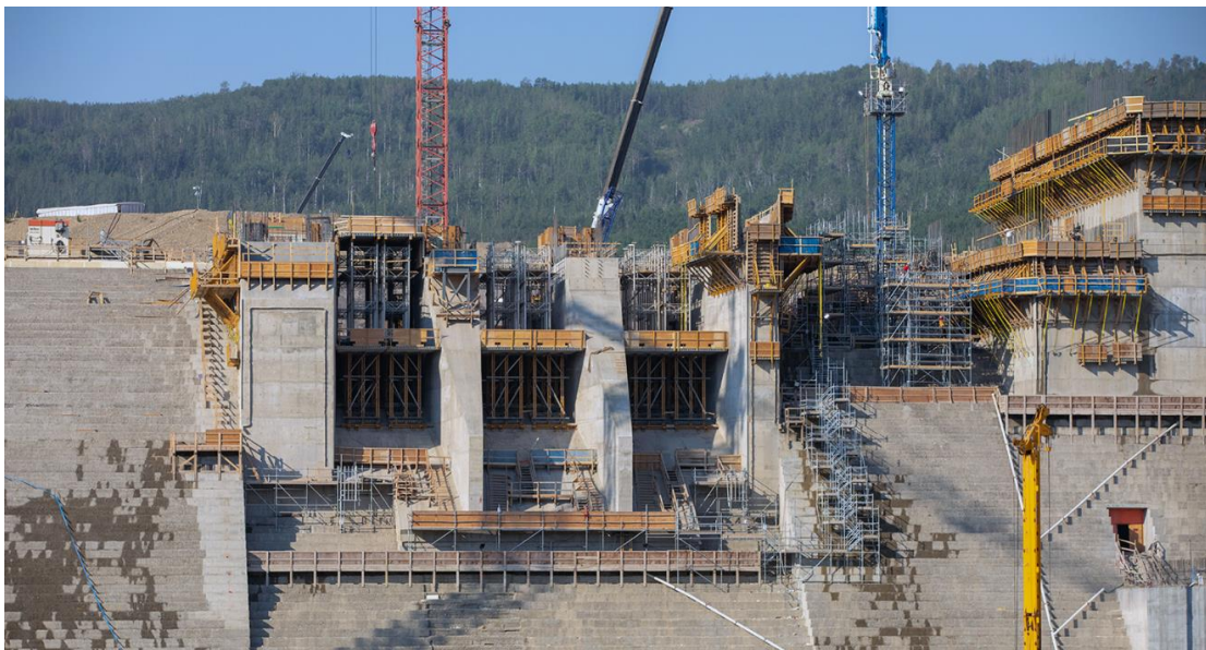
Figure A-4 Construction progresses at the spillway headworks east low-level outlet gate. The spillway will allow the passage of large volumes of water from the reservoir into the river channel downstream (July 2021)
