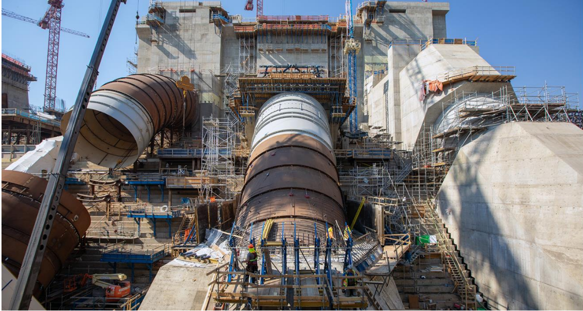
Figure A-3 Penstocks for units 1, 2 and 3 (July 2021)
