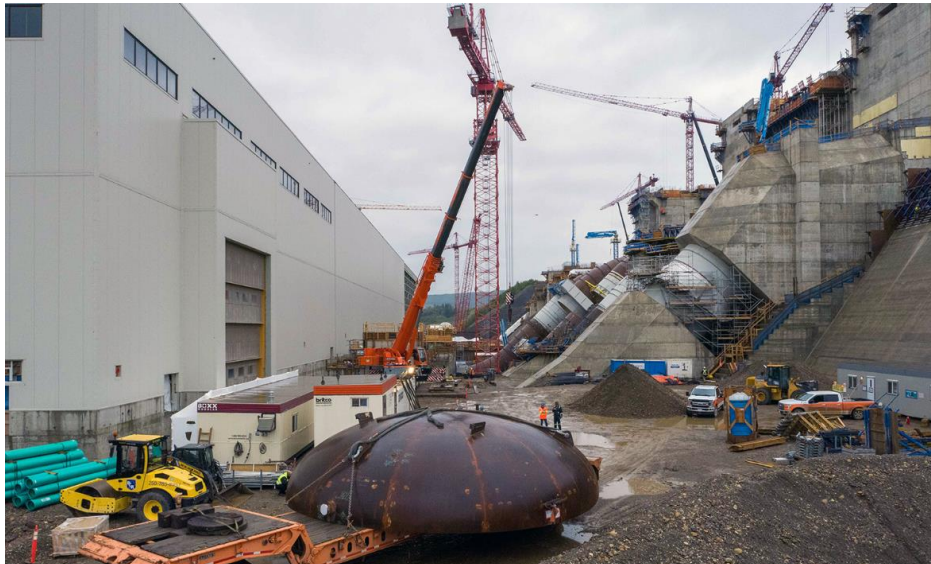
Figure A-6 The first of four spiral case inlet bulkheads is delivered from the Voith warehouse at site to the powerhouse (August 2021)
