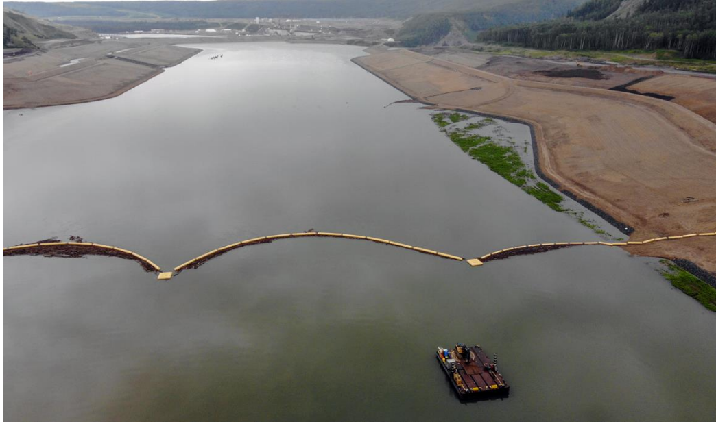
Figure A-1 An aerial view of the headpond and debris boom where a barge is used for clearing debris materials from the boom (July 2021)
