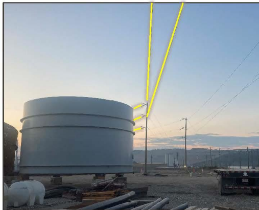
Figure 5 A section of penstock stored adjacent to a high voltage conductor.
