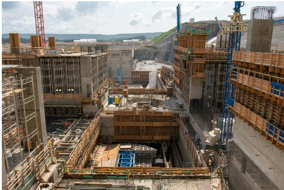
Figure A-2 Construction Continues on the Powerhouse (July 2019)
