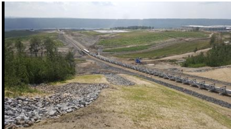
Figure A-9 The 5km Conveyor System, which Runs from the 85 th Avenue Industrial Lands to the Dam Site, will Carry Glacial Till, an Impervious Clay-like Material that will Form the Core of the Dam. The Conveyor System was Chosen as the Primary Form of Transport because it will Reduce Traffic on Local Roads, Create Fewer Greenhouse Gas Emissions, and Result in Less Noise and Dust (September 2019)
