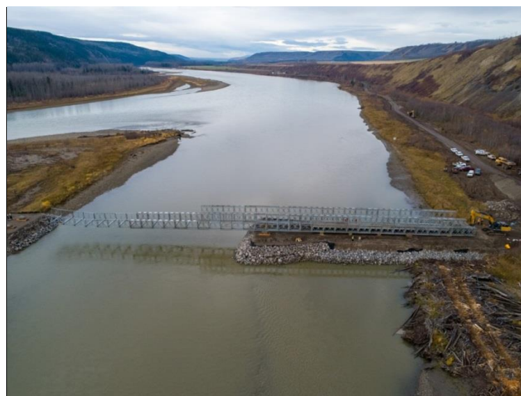
Figure A-10 Construction Started on a Temporary Bridge to an Island in the Peace River near Halfway River, as Part of Clearing Activities for the Project. The Bridge allows Workers to Remove Vegetation from the Island and Prepare for the Creation of the New Reservoir (September 2019)
