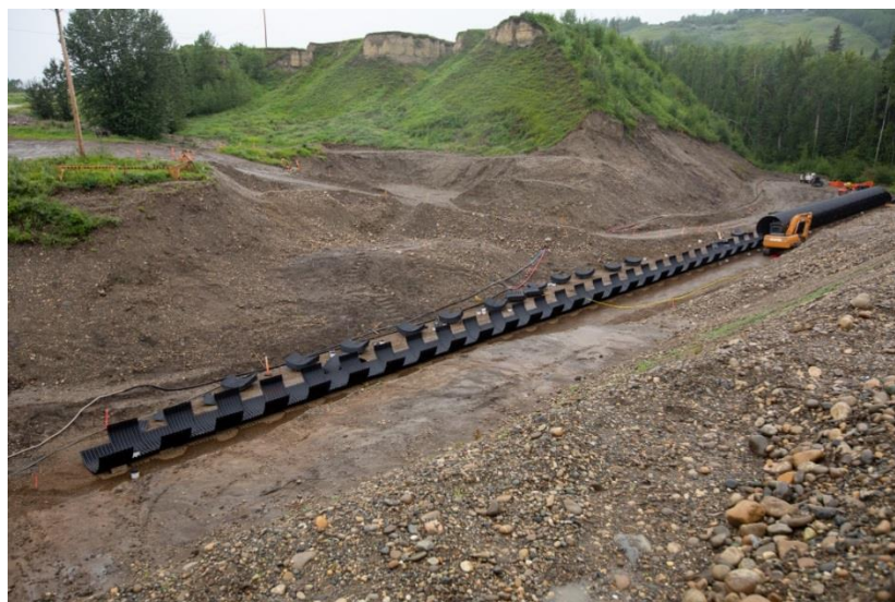
Figure A-4 Assembly of a Multi-plate Culvert that will Provide Drainage under a Realigned Segment of Highway 29 in the Cache Creek Area. A variety of Culverts are being Installed as Part of the Highway 29 Realignment (July 2019)
