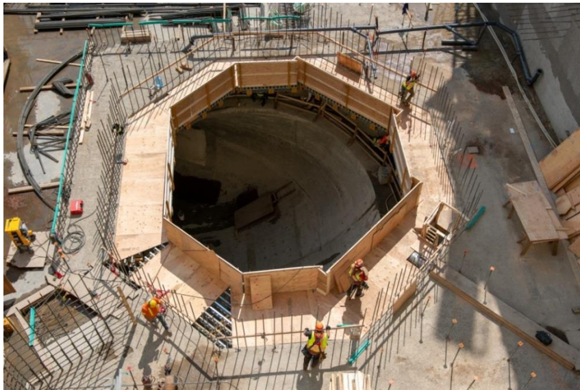
Figure A-3 View of Inside Unit 1 Draft Tube in the Powerhouse. Once Site C is Operational, Water will Enter the Penstocks, Move through the Turbines and Generators and then be Released into the Draft Tubes prior to Exiting through the Tail Race (July 2019)
