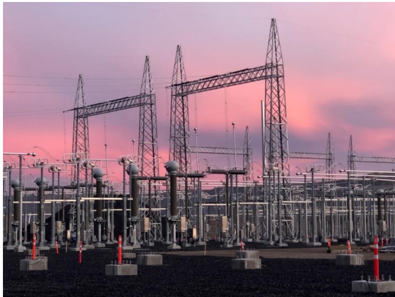
Figure A-6 The Site C Substation will be the Largest in BC Hydro's System. The Substation is 80 per cent Complete and Scheduled to go into Service in October 2020 (August 2019)
