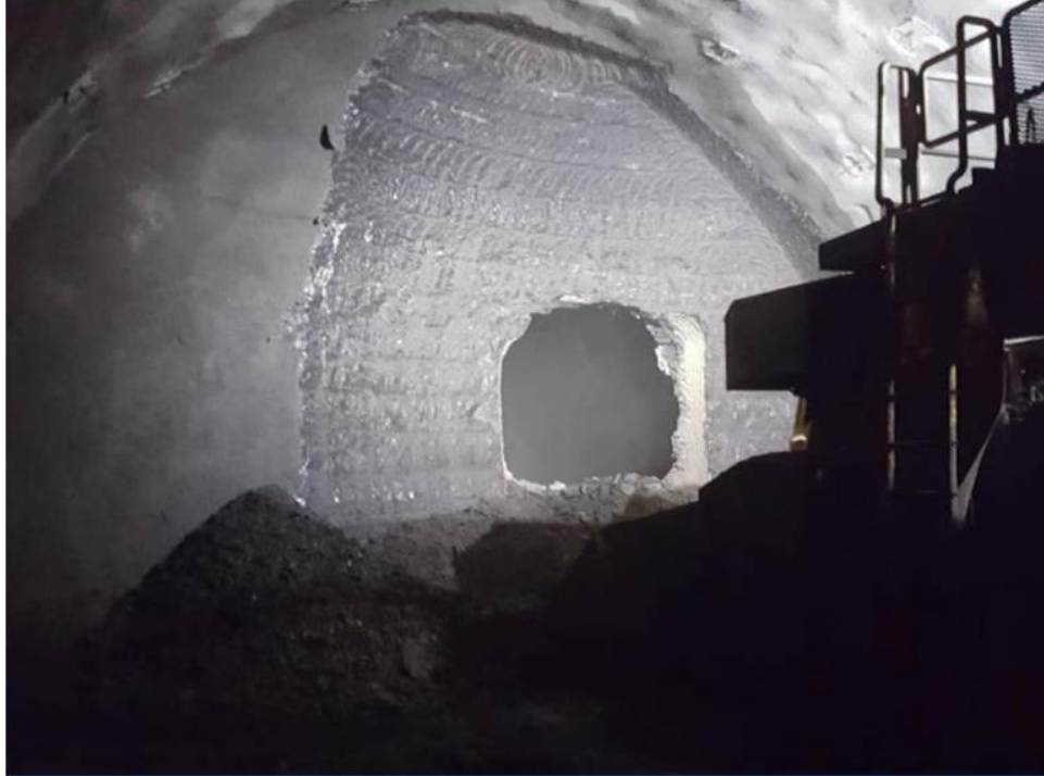
Figure A-1 Diversion Tunnel No. 2 Breakthrough (July 2019)
