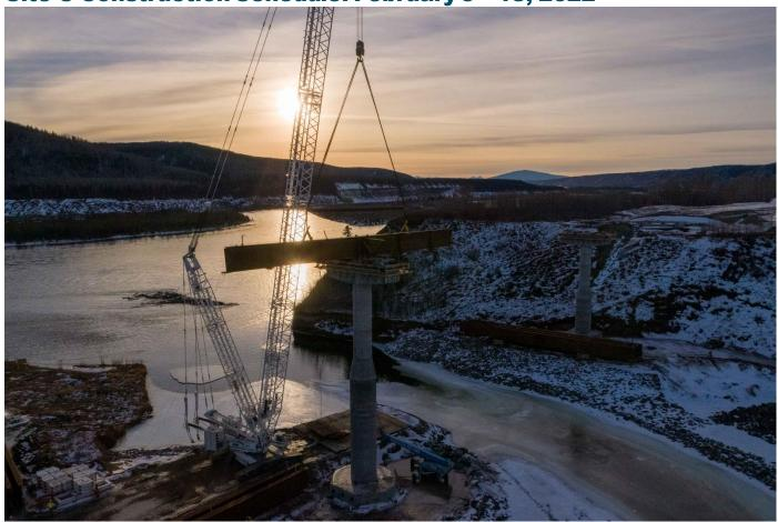
Crews lifting and installing the girders across the new Farrell Creek Bridge. It is one of five new crossings along Highway 29, and completion is expected in 2022. More photos in the <u>image gallery</u>.
