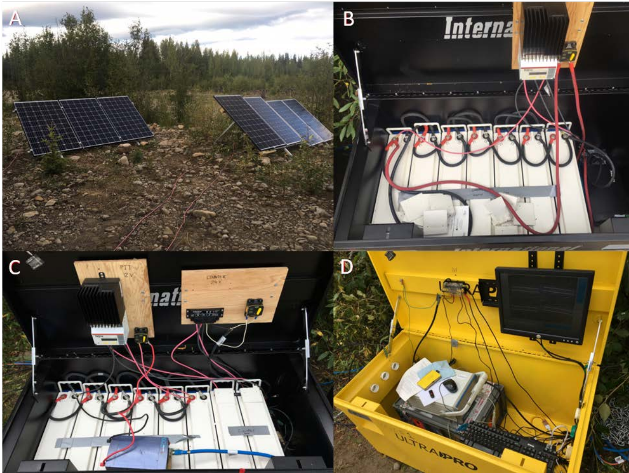
Figure 2. Power system configurations used in the Chowade River and Cypress Creek, 2017. Panel A shows the solar panel setup, panel B depicts the video validation and computer battery bank, panel C depicts the battery bank used for the resistivity counters and PIT arrays, and panel D depicts the resistivity counter and computer/DVR system.
