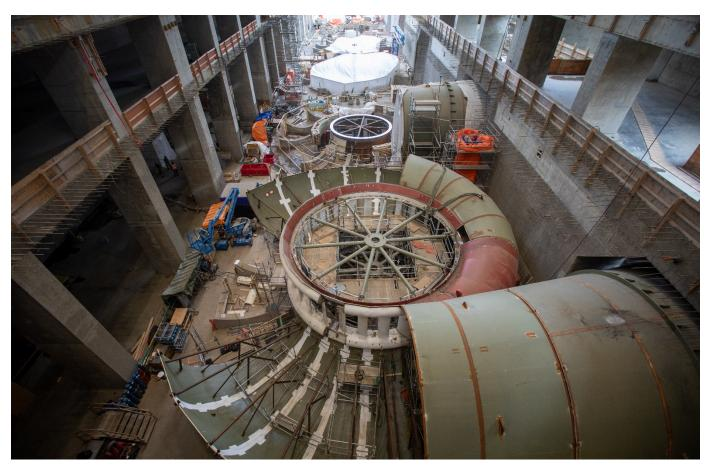
Installation of the thrust rings and spiral casings at penstock Units 1 and 2 is underway. The items are part of the turbineembedded components for Units 1 and 2 inside the powerhouse. See more project photos in the image gallery.
