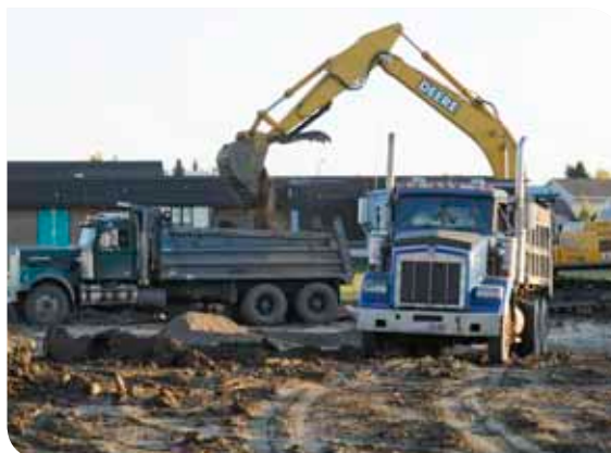
Construction project in Fort St. John.
