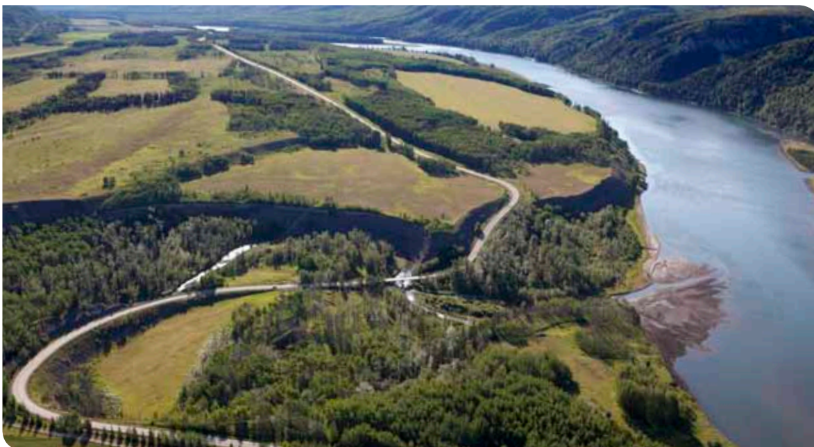
Highway 29 at Farrell Creek.
