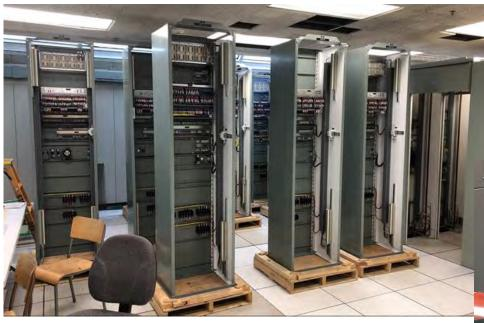
New protection panels ready for installation in Peace Canyon control room and wiring to the new Protection & Control panels
