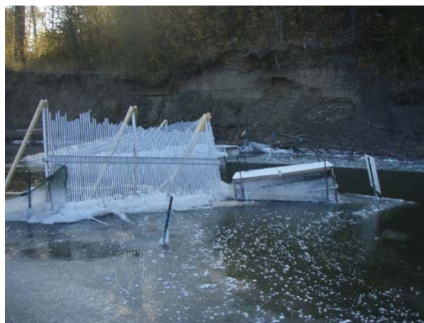
Plate 5: Ice damming at the fish fence on the Moberly River, fall 2009.
