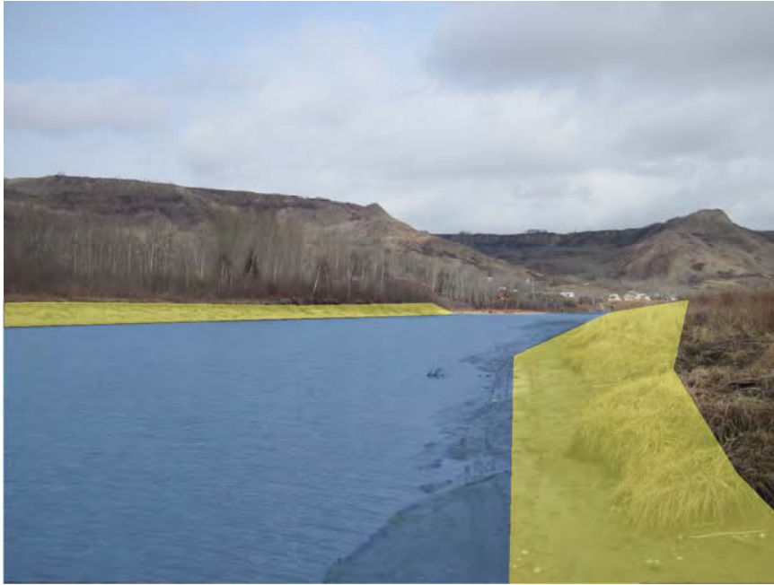
Photo 3. South arm side channel at 109L. View looking downstream (east) from inlet at main channel. Preliminary design works includes deepening the existing channel and re-contour the bankline. Excavated material will be side cast on bank. Yellow shading estimates fill and blue shading estimate cut extents.
