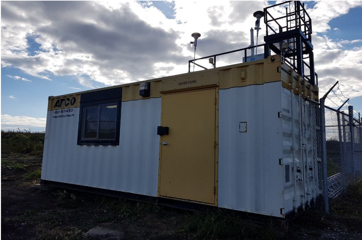
Figure 2-4: Upgraded Station 9 (85th Avenue)
