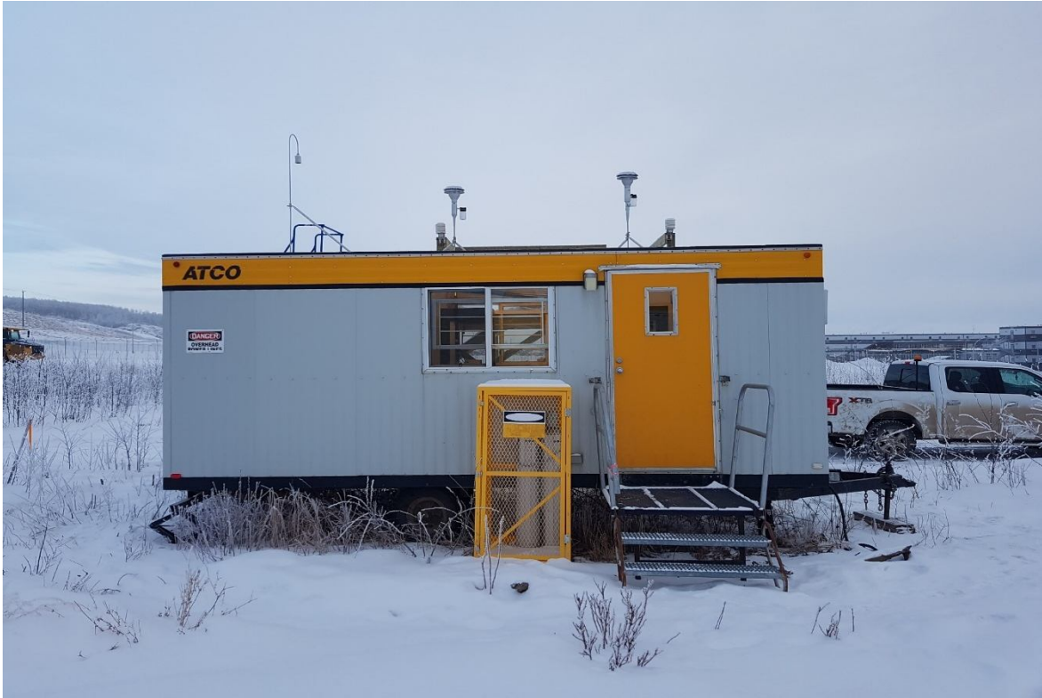
Figure 2-3: Upgraded Station 7B/C (Site C North Camp/Fort St John Camp C)
